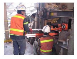
Belt Cleaner technicians from P.T. Suprabakti Mandiri (Supra) install a Martin Engineering secondary cleaner on a conveyor at PTFI.
