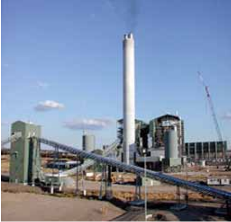
Coal-handling conveyors at the new Millmerran Power facility incorporate belt cleaners supplied by Martin Engineering's Australian licensee.
