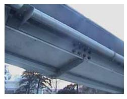
The air supported conveyors in the Coors Brewing Company plant in Golden, Colorado incorporate air-supported returns to eliminate idler bearings and the maintenance they require.
