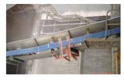
The Martin® Air Supported Conveyor installed at Cementos Progreso was engineered with a vertical curve in the center third of the conveyor's 156-foot (47.4-m) length.
