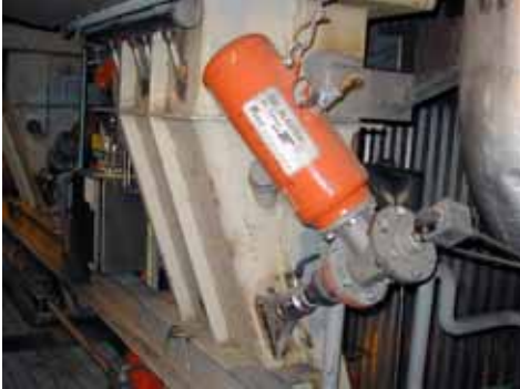
Martin® Air Cannons were installed to prevent choking of pet coke feed chutes at the Bay Shore Power Station.
