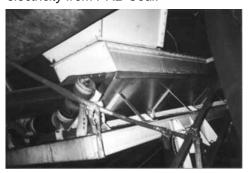
To improve its performance, the power plant converted the initial seventy feet (21 m) of the S-2 Conveyor to the Martin® Air Supported Conveyor System.
