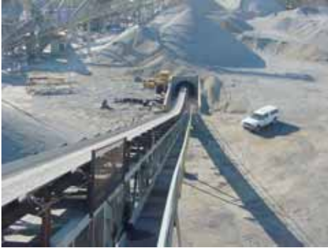
Conveyors at this Georgia quarry suffered from high amounts of carryback.
