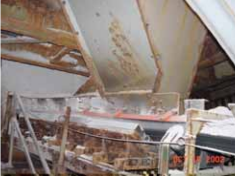
Martin® Self Adjusting Skirting is installed on a conveyor at Morton Salt in Grand River, Ohio.
