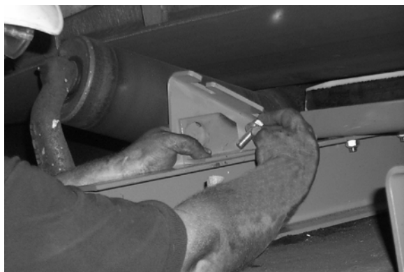
15. Bolt on the fine tune adjustment angle but do not tighten.
