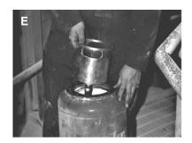
4. Remove existing piston/cylinder mechanism from tank (E).
