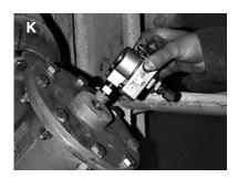
10. Apply thread sealant compound to both ends of nipple and install in QEV. Install QEV into rear of valve assembly with exhaust port pointing down and away from personnel (K).
