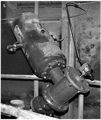
11. Connect existing air supply to QEV inlet port and re-install safety cable (L).
