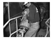
3. Remove safety cable (B) and quick exhaust valve (QEV) (C) (if present) from existing air cannon. Remove existing cannon from its mount (D). (IMPORTANT: Martin Engineering recommends using QEV P/N 18858 with Martin<sup>®</sup> XHV Retrofit Valve.)
