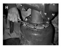
7. Position valve assembly over gasket and secure with fasteners (H). Tighten to snug.
