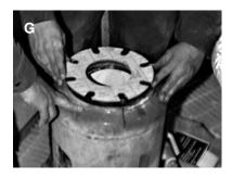
6. Position supplied gasket on tank flange (G).
